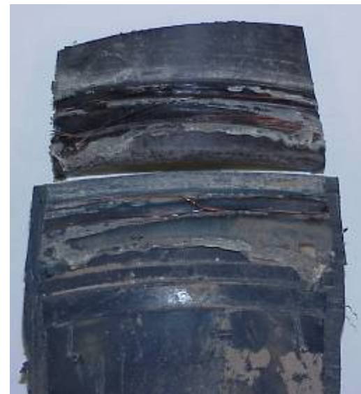
Pipe and fitting were not cleaned!
